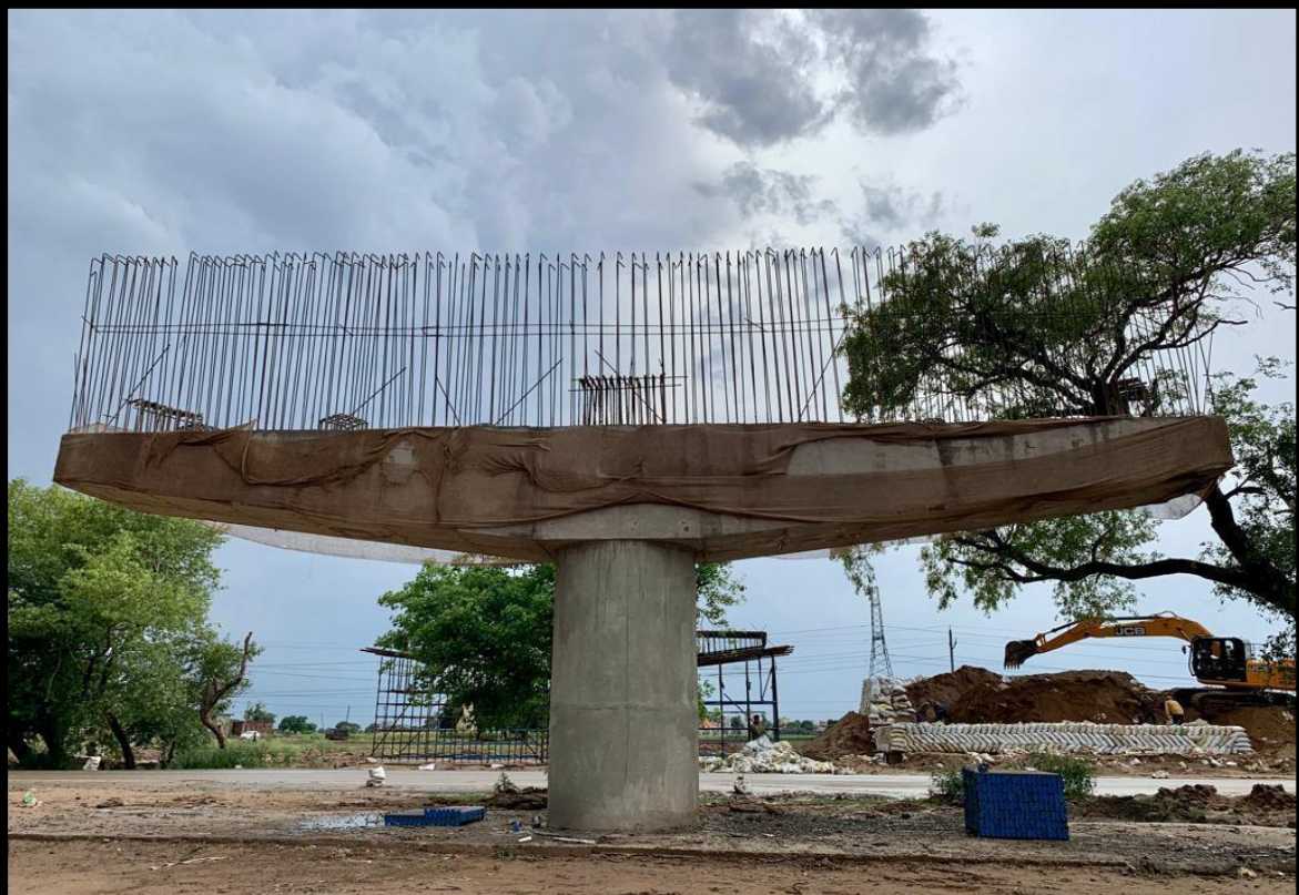
Abutment (A2) of Flyover @ Ch:9+270
