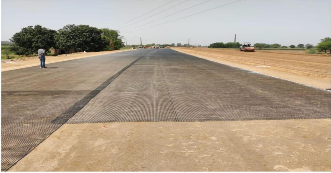
GEO-GRID LAYING @ Chainage 81+850 to 82+100
