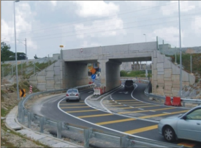
Completed Structure RUB
