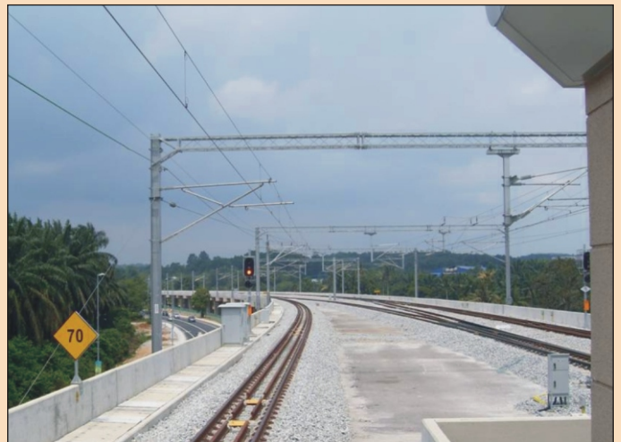
Completed Viaduct In Phase-1
