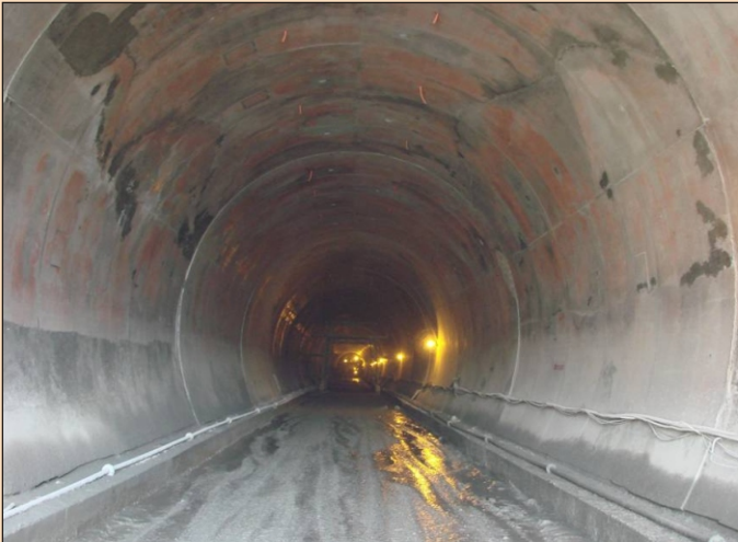
Finished Tunnel Lining of T - 80
