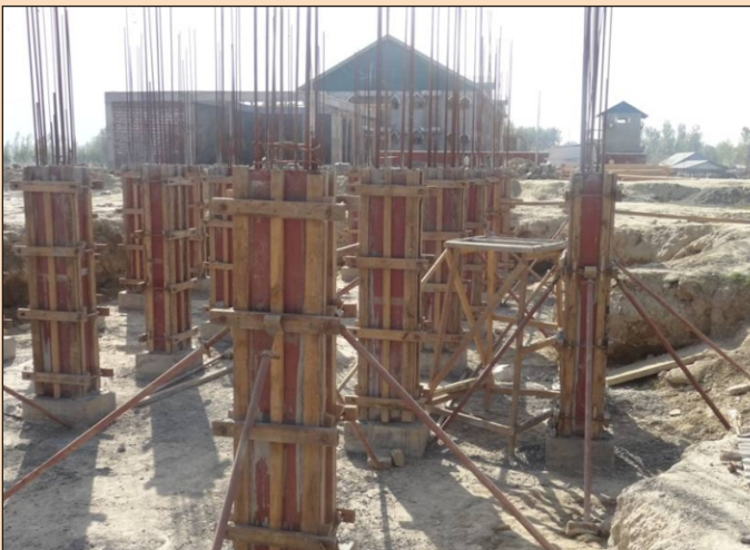
Railway Staff Quarters Work in Progress at Srinagar
