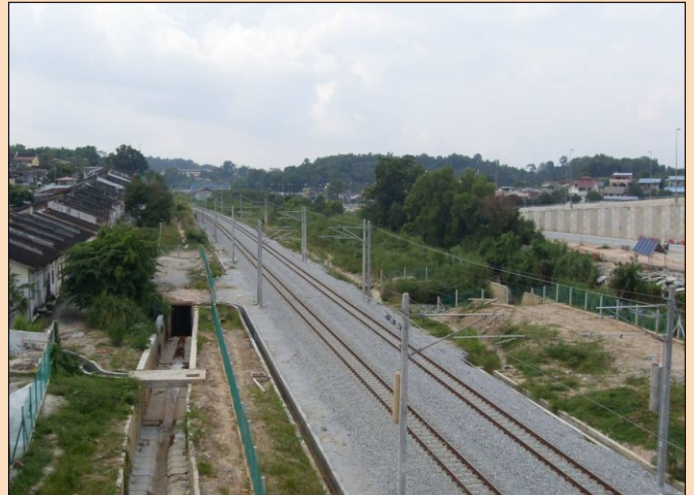
Commissioned Track With Electrification Works
