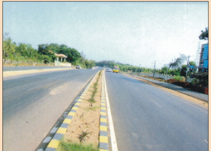
Port Connectivity road project Manglore
