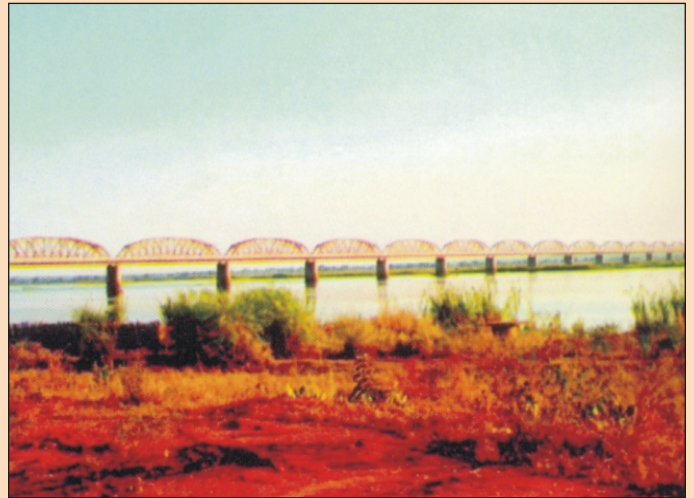
Rehabilitation of DONA ANA Bridge in Mozambique
