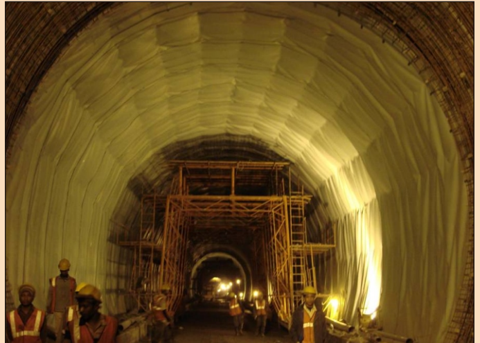
Water Proofing Membrane Installation in T - 80
