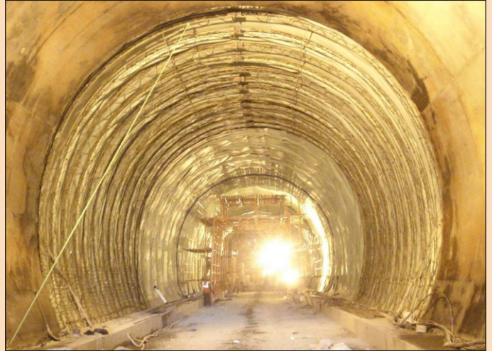
Lining Works T - 80
