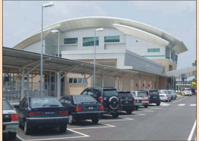
View Senawang Station Building
